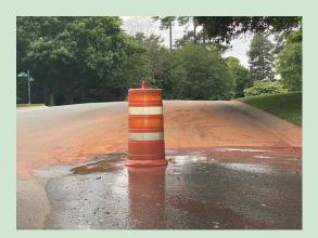
The water line break under Harbor Light (near the intersection with Jetton Road) is creating a sink hole under the pavement.
